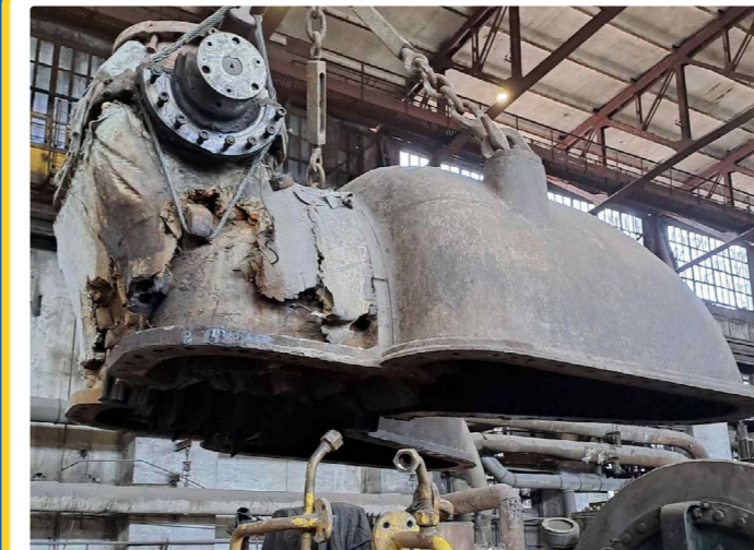
Major overhaul work for the power unit machinery at Unit 4 at CHP owned by Kamet Steel PrJSC, Metinvestholding, including turbine AT-25-2 ТМ3, generator ТГВ-25, pumps, condenser, heaters and other machinery for the turbine hall; repair work for the electric motors for pumps and other systems, replacement for high-voltage circuit breakers, repair work for other electric equipment and I&C.
