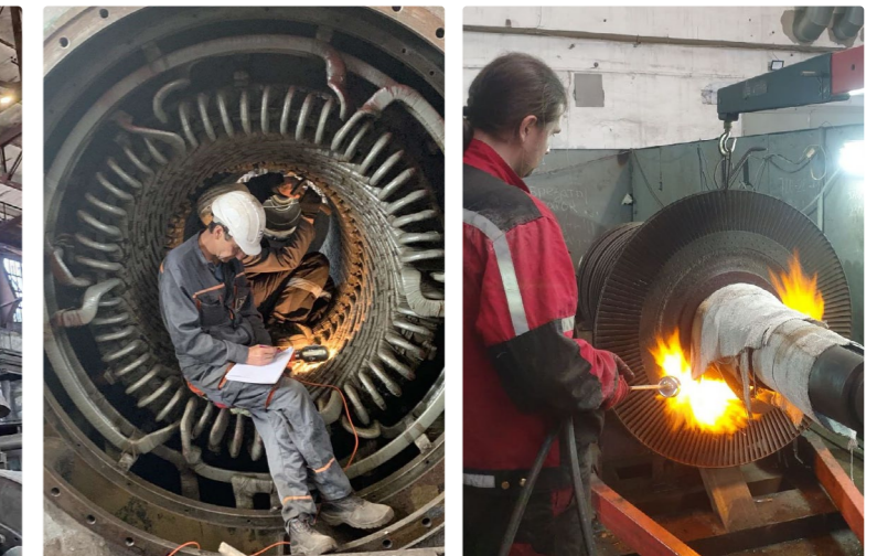
Major overhaul work for the power unit machinery at Unit 4 at CHP owned by Kamet Steel PrJSC, Metinvestholding, including turbine AT-25-2 ТМ3, generator ТГВ-25, pumps, condenser, heaters and other machinery for the turbine hall; repair work for the electric motors for pumps and other systems, replacement for high-voltage circuit breakers, repair work for other electric equipment and I&C.
