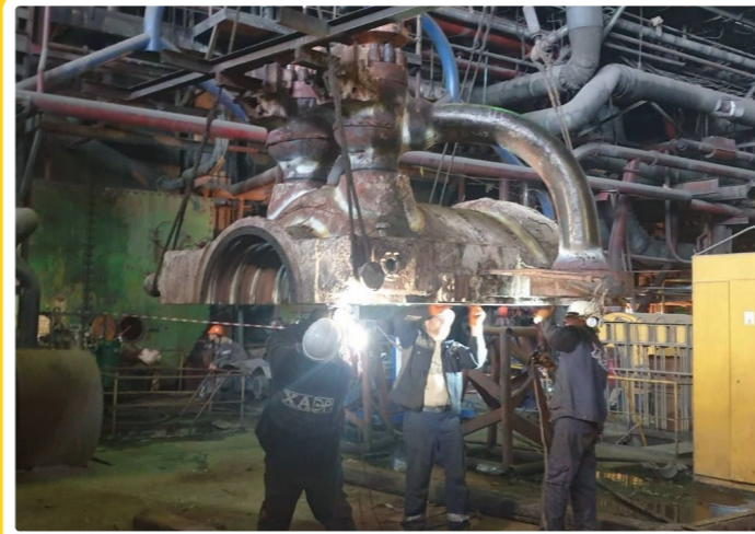
Repair work for the K-200-130 turbine, Unit 9, and repair work for the high-pressure cylinder the intermediate-pressure rotor with replacement of damaged blades and turbine shrouding of the K-200-130 turbine, Unit 7, at DTEK Burshtyn TPP, Zakhidenergo.
