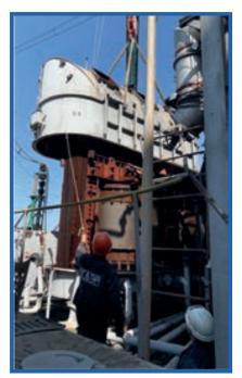
A separate area of work performed by the Electric Department is to overhaul transformers of voltage classes from 6 kV to 750 kV and with a power rating from 1 MVA to 1250 MVA.
