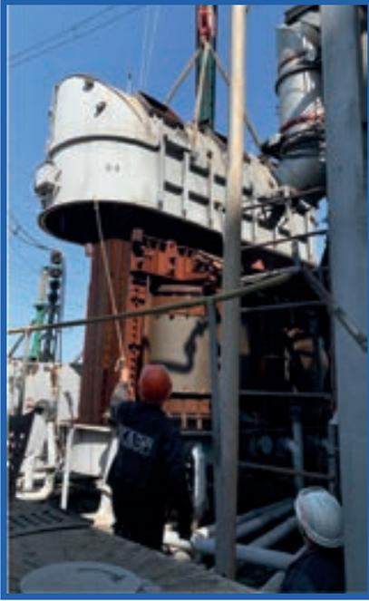
A separate area of work performed by the Electric Department is to overhaul transformers of voltage classes from 6 kV to 750 kV and with a power rating from 1 MVA to 1250 MVA.
